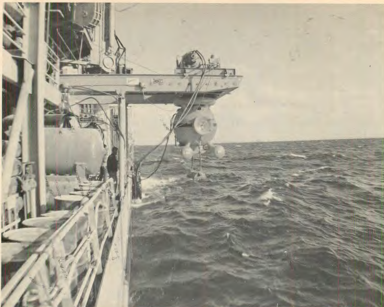
A diving bell (center) ready to be lowered over the side of an underwater-pipeline laying barge. The deck decompression chamber, or DDC, is at left.
