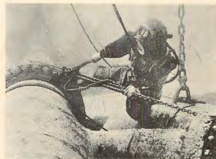
A diver with surface air supply
