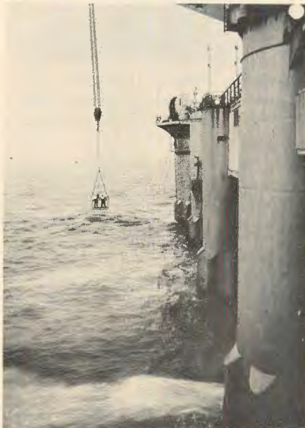
Two divers wearing SCUBA (self-contained underwater breathing apparatus) being lowered over the side of a huge semisubmersible North Sea oil rig
