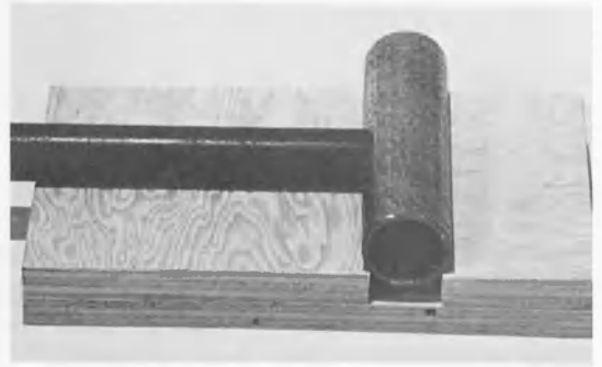
Fig. 6 -- At A, the spider welding fixture is constructed on a 2 foot x 2 foot x 3/4-inch plywood base. Evenly spaced 5 3/16-inch x 16-inch ramps provide the 18-degree spreader angles. At B, a hub axle and mast T fixture lifts the 1-8 inch mast pipe for welding at right angles to the 1-1/2-inch axle pipe.
