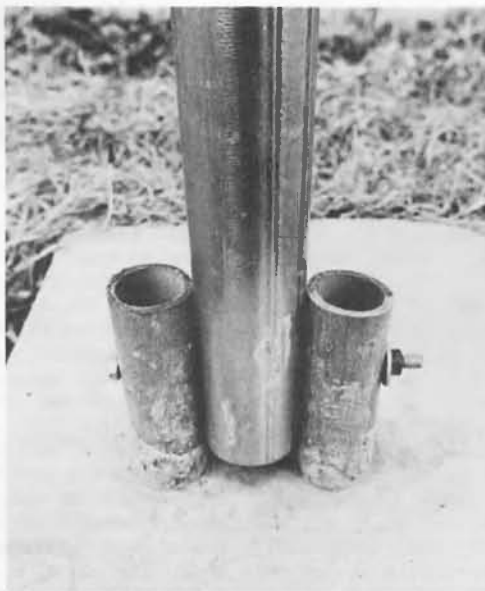
Fig. 2 -- A mast hinge is made of two lengths of 1-1/2-in iron pipe set in concrete. Their 1-3/4-in separation accommodates the steel conduit of the homemade telescoping mast.
