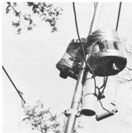
Fig. 10 — Freezer jars weatherproof the gamma capacitors.
