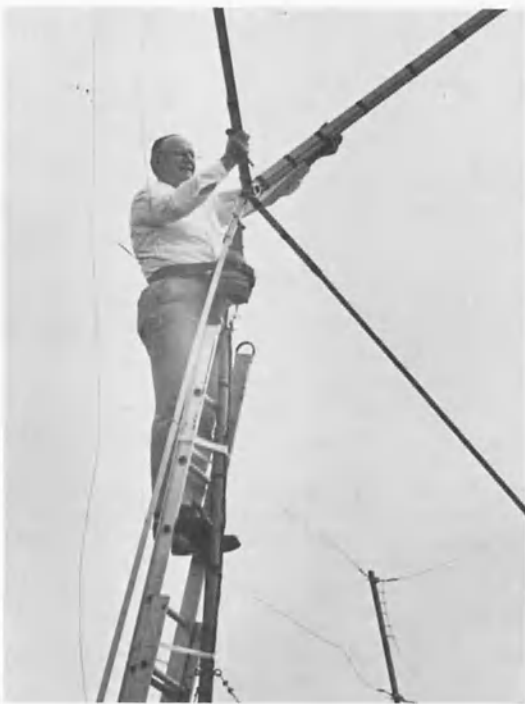
Fig. 4 -- NØARQ slips the reflector element onto the mast T. A 63-inch spruce tie bar supports 12-inch x 3-inch mini-stubs in the bottom center of each reflector loop.
